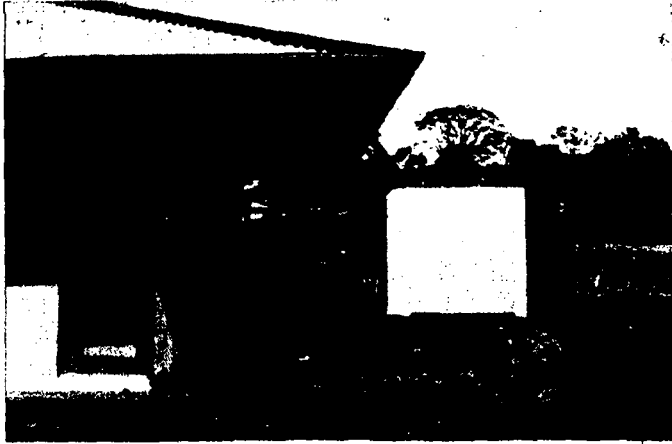
Photo 1 A cistern and a well for water supply constructed on project site.
