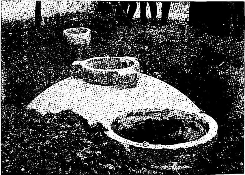
Fig. 18: Dome biogas plant. The inlet, the dome cover opening and the discharge shaft are clearly visible. Once the plant has been finished, only the shaft cover remains visible.
