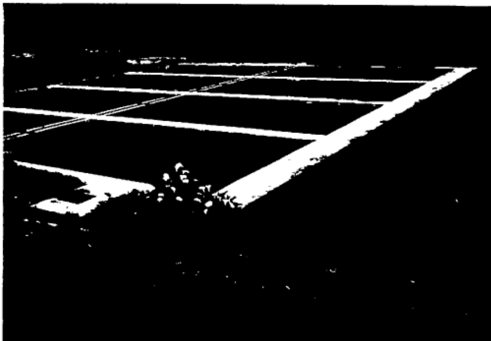
Figure 19. Sludge drying beds.
