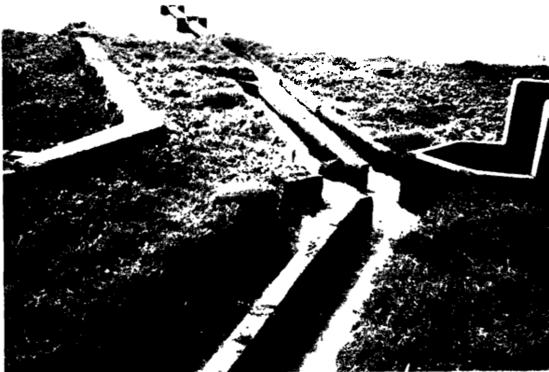
FIGURE 23. FLOW DIVIDING POINT AT THE MINDOLO PONDS.
