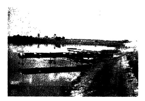
Fig. 7.17 **Outlet structure on final maturation** pond at the line A before it filled up after remedial work was done. Note the paving slabs are in place.
