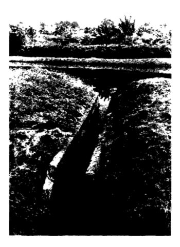
Fig. 7.7 Maturation pond outlet Note that flow is just a trickle
