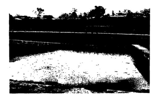
Fig. 7.3 showing scum baffle and scum which has accumulated at the inlet of primary pond
