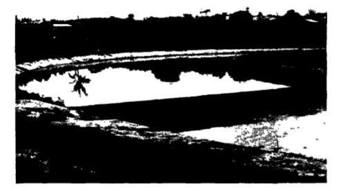
Fig. 5.1 Circular Waste Stabilization Pond
