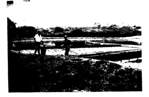
Fig. 7.5 workmen removing scum using dippers at Embu
