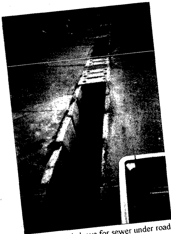
Plate 1. Excavation for shallow sewers.
