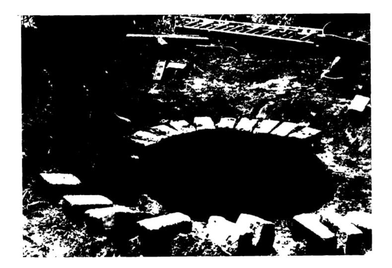
Figure D. Laying the brick collar.
