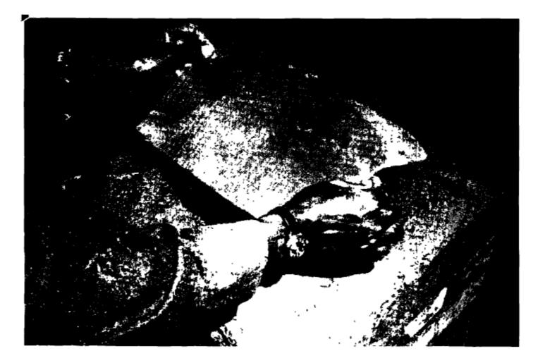
Figure M. Flyscreen mortared to top course of brick vent pipe.
