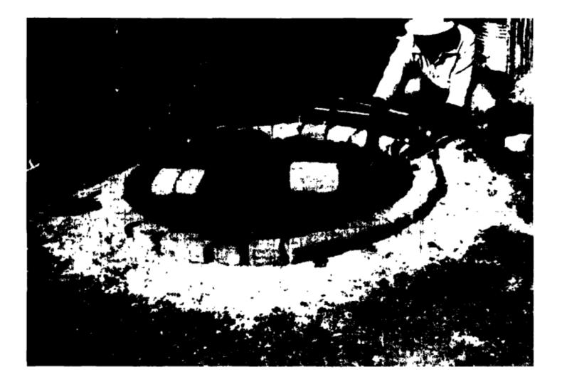
Figure E. Casting the reinforced concrete coverslab on site.
