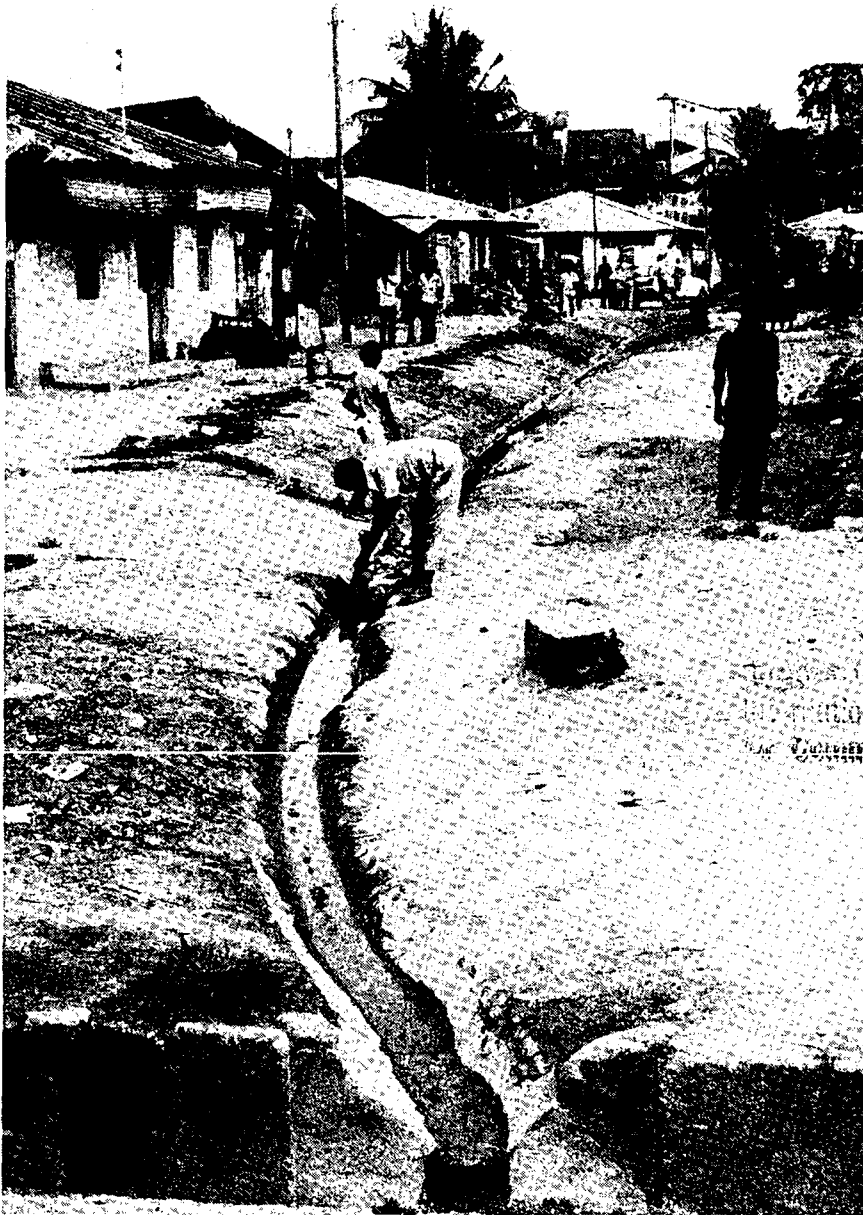
Open drains provide places for insect breeding as well as allowing access to polluted waste water for children and animals
