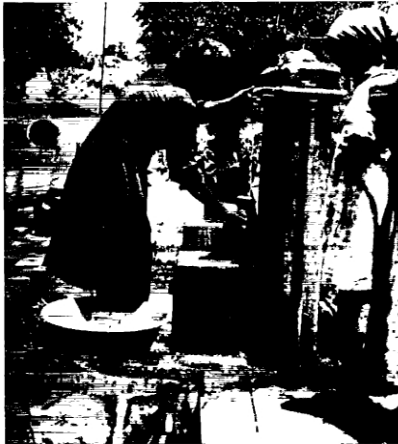
Figure 6. Self-closing "Talflo" trap installed on a public standpipe. 21
