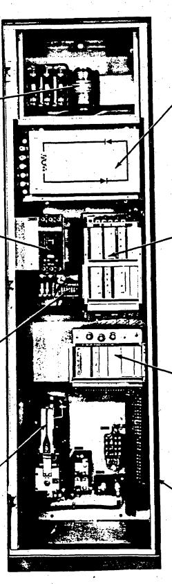
**CONVERSION MODULE** – A single drawout assembly of 6 SCR units (individually removable) in a full 6-way bridge. SCR protective devices and feedback circuits are an integral part of the assembly.
