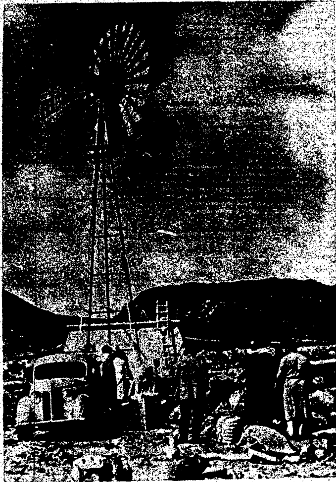
Fig. 31 (a) - Hercules water pumping windmill (By courtesy of H.J. Godwin, Ltd.)
