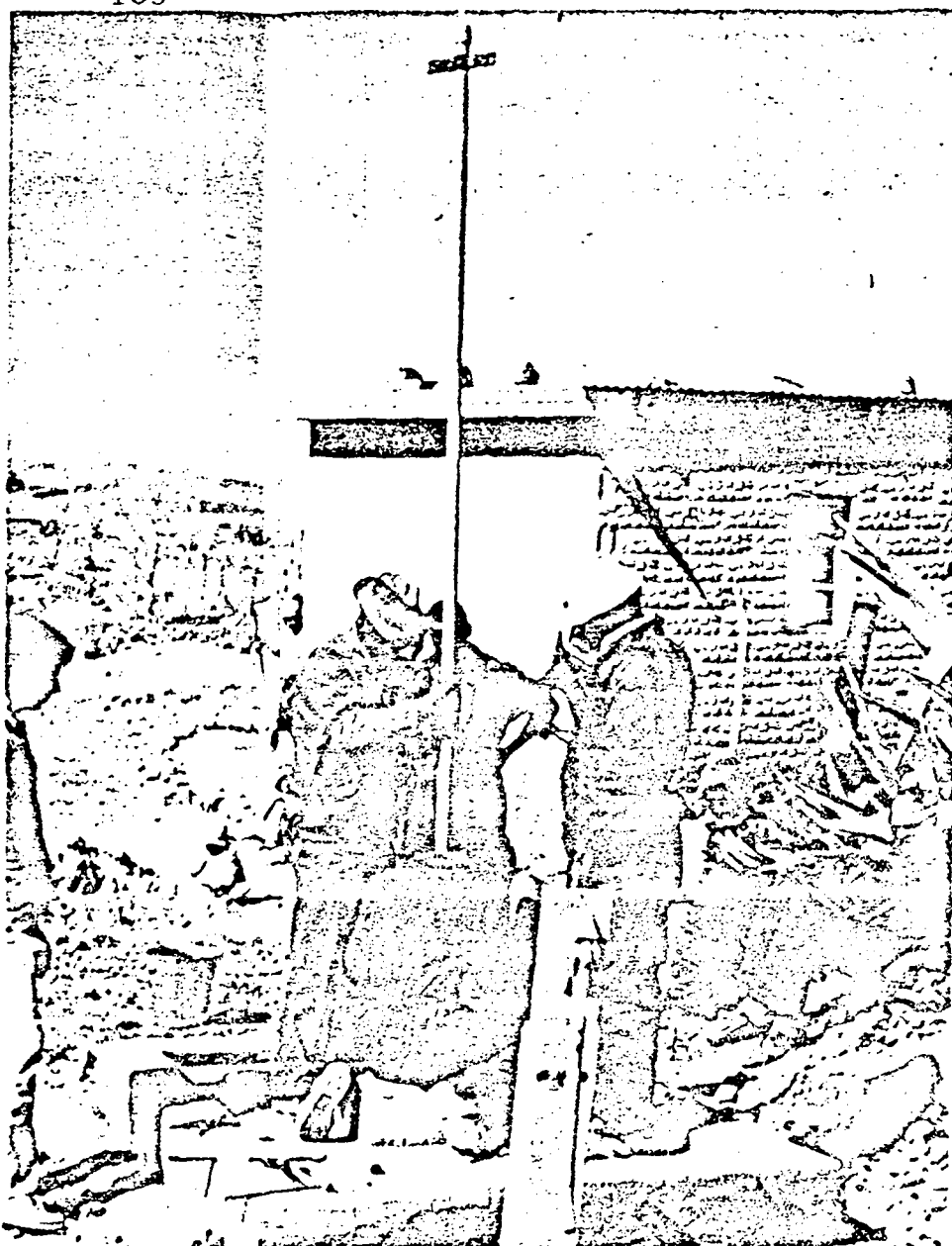
The Consallen's plastic drop-pipe makes installation and removal of the underground equipment a simple operation (above). The completed installation (below) is the closest currently available to the UN panel's VLOM pump ideal.
