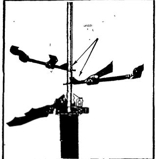
KEEP ON LOWERING THE PIPE AND CONNECTING ROD INTO THE BORE/TUBE WELL TILL THE LAST PIPE.
