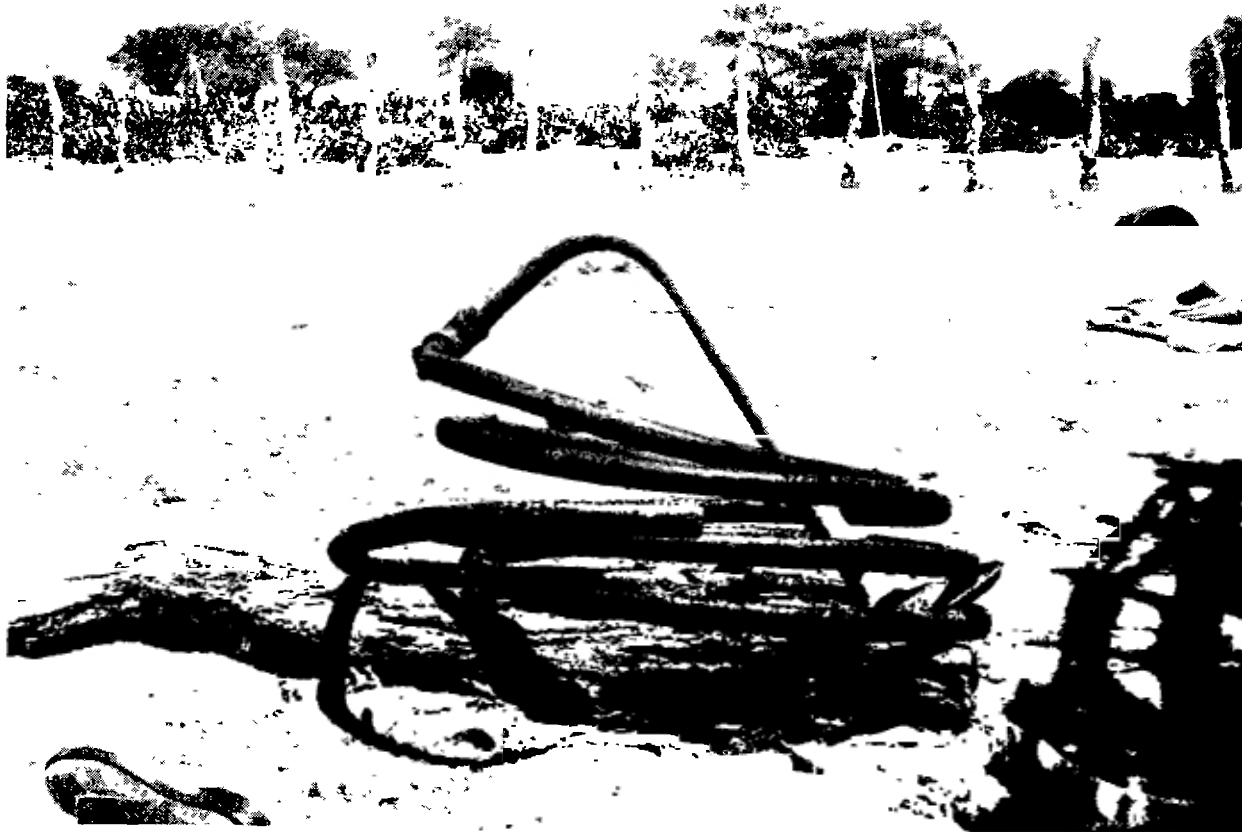
Photo 4. Picture of a destroyed Copper Coil at Mathathane.
