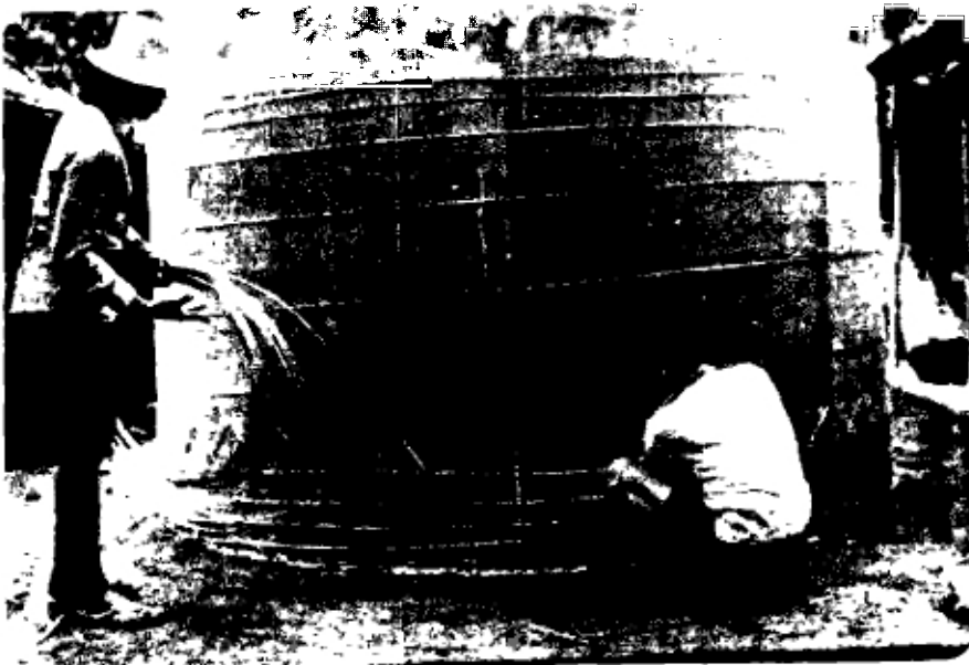
PHOTO 33: THE SECOND LAYER OF IRON WIRE IS WOUND AROUND.
