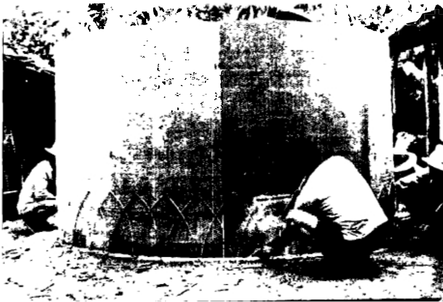
PHOTO 24: AND THE CROSSINGS ARE FASTENED TO THE CHICKEN WIRE.
