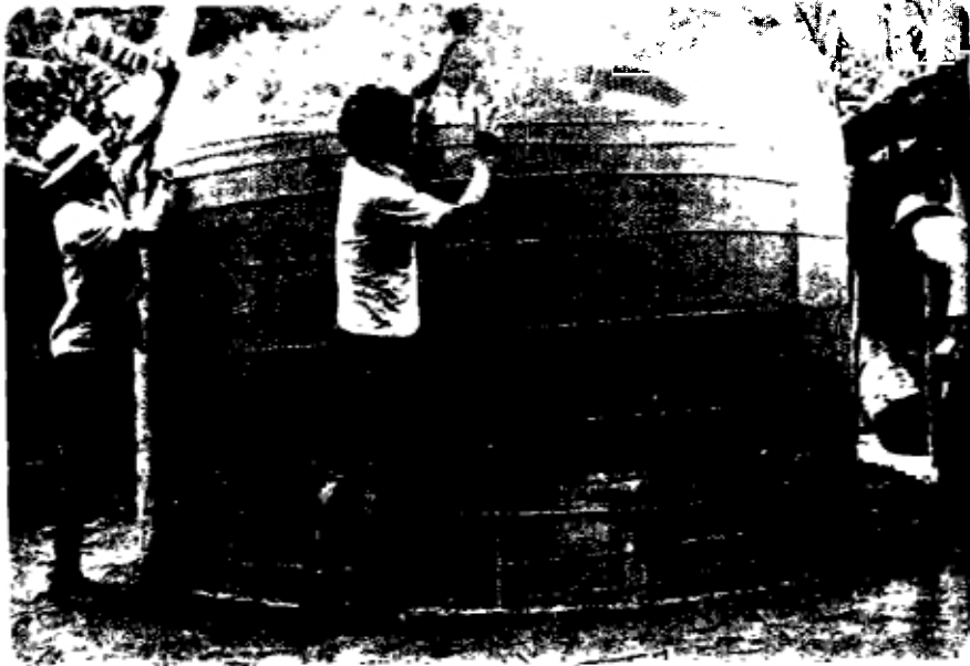
PHOTO 32: THE SECOND LAYER OF CHICKEN WIRE IS ATTACHED WITH A 30cm OVERLAP ABOVE THE MOULD.
