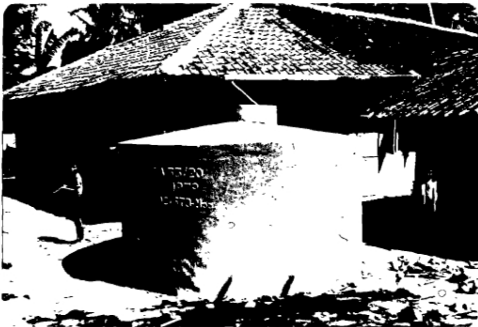
PHOTO 56: RESERVOIR READY FOR USE.
