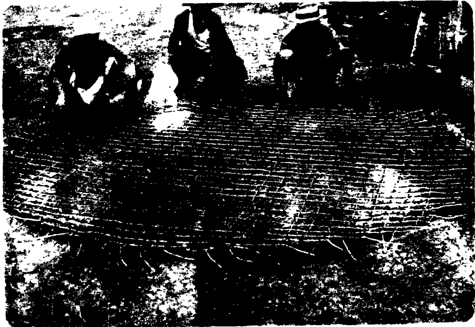
PHOTO 43: REINFORCEMENT FOR THE ROOF.
