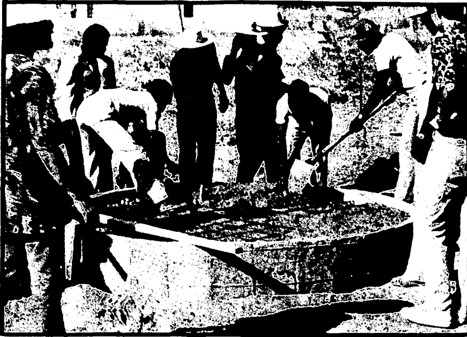
Photo 1. Trainees pouring the reinforced foundation of the cistern.
