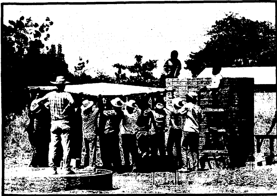
Photo 5. Trainees hoist the formwork to pour the cistern's cover slab in place.
