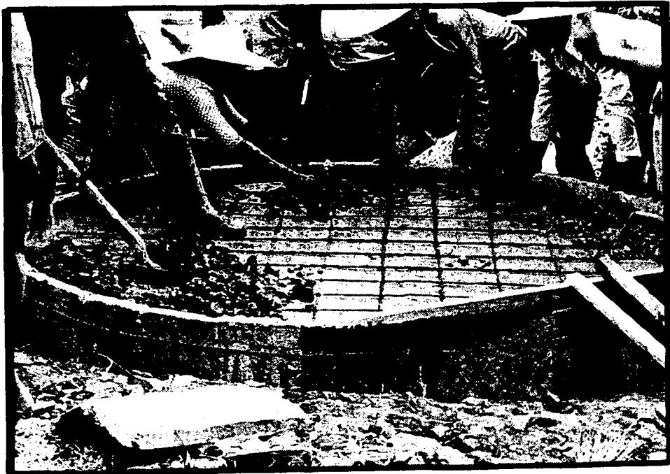
Photo 6. Trainees cementing the cistern drain and faucet.
