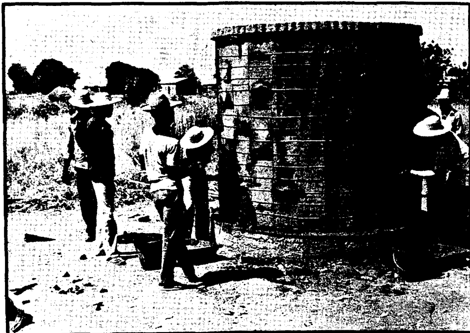
Photo 8. Trainees beginning to apply the exterior layer of mortar to the cistern.
