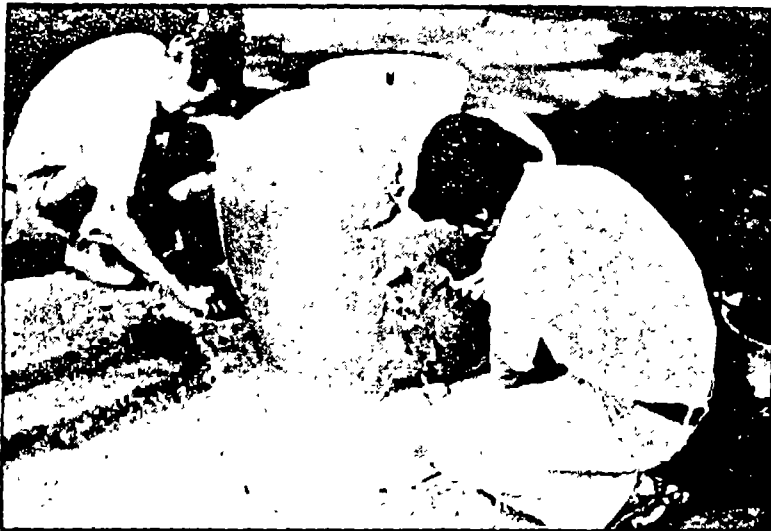
2.8 Trowel a first layer of mortar onto the mould to a thickness of about 0.5cm.
