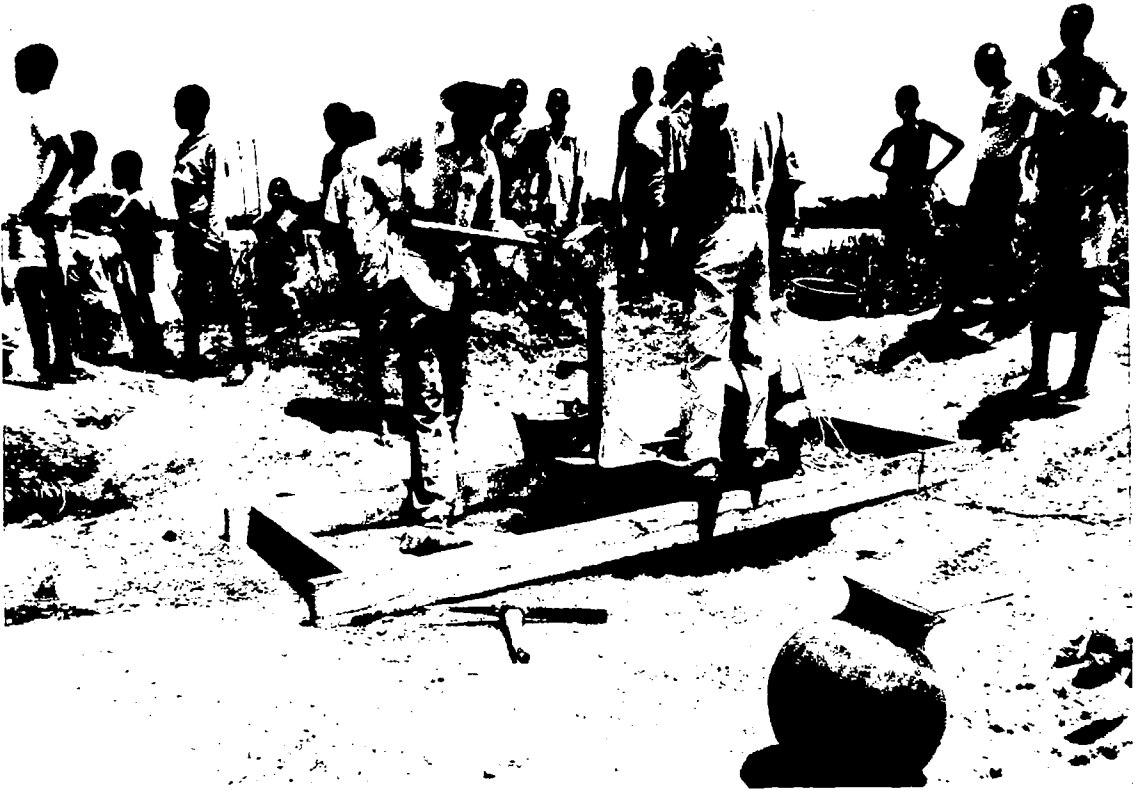
A SWN 80 pump used for dewatering a hand-dug well.
