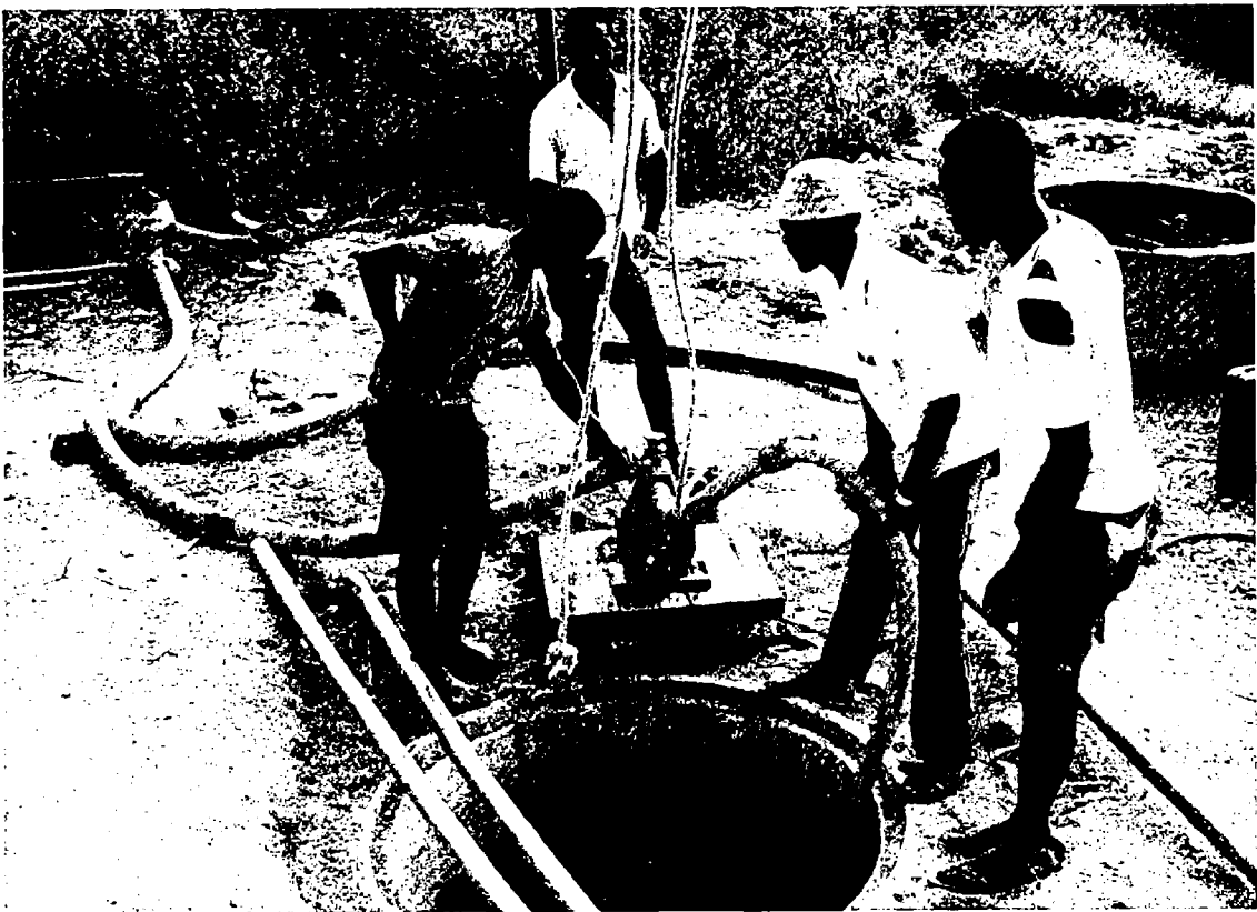
Excessive inflow of groundwater necessitates the use of motor pumps
