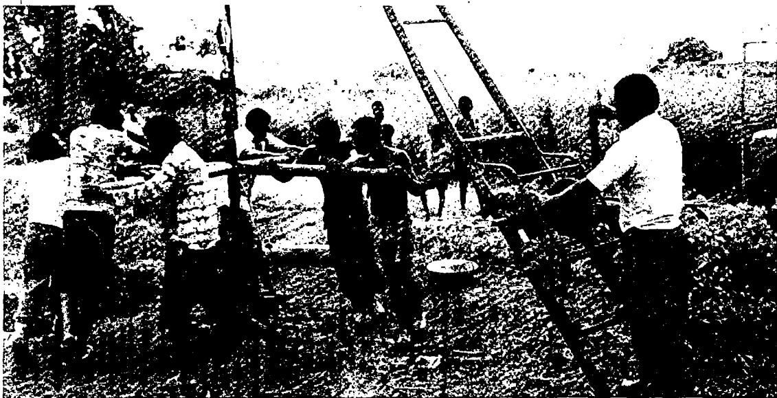
Hand-drilling in progress
