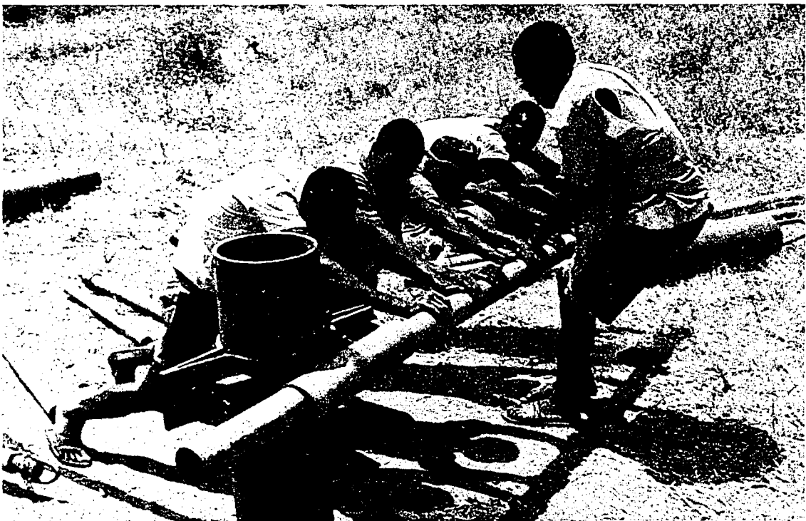
Pressing down the casing
