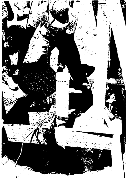
Pouring of gravel around the PVC filter
