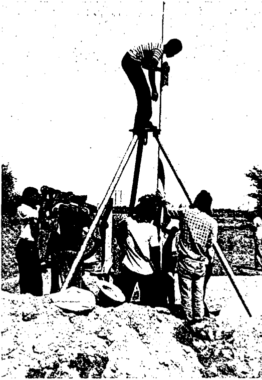
Installation of the string of PVC
