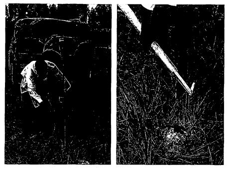
23. The casing is lowered by turning and pressing it downward when the bailer is lifted
