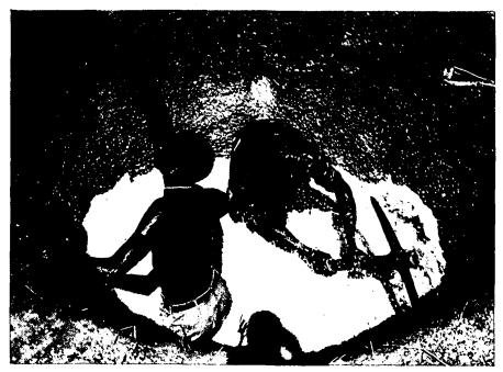
44. Well with excessive recharge. Two pumps are used to remove the water (see suction hoses at left)
