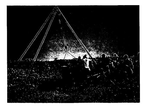
49. The ring is hoisted into position over the well
