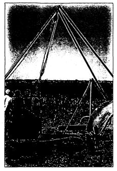
45. A concrete ring is rolled to the well and the 5.50 m sling is fastened around it. The tripod is positioned next to the well opening
