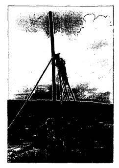
72. The filter pipe is lowered in the borehole
