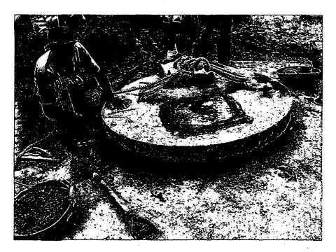
55. A watertight connection is made between well rings and cover
