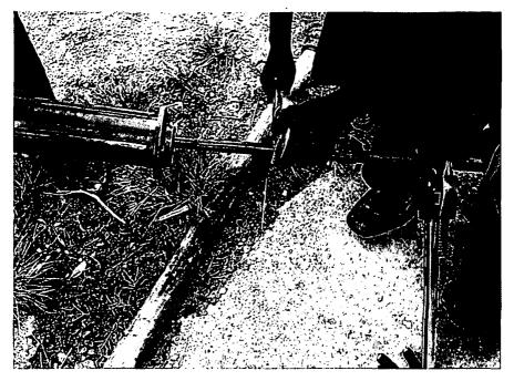
119. An extension rod is connected to the pump rod
