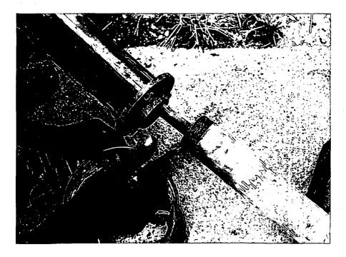
120. Bituminous paint is applied to the thread of the rising main
