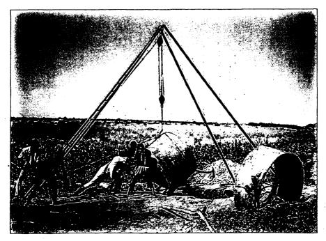
47. The bottom of the ring is pushed towards the well edge and the tackle rope is paid out, until the rings rests on the ground in horizontal position
