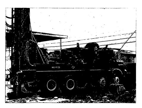
81. Heavy motor-driven rotary drill
