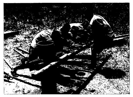
66. A casing pipe is screwed into the soil
