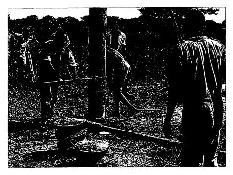
78. Section-wise removal of the casing. Note the 'karai' with filter material on the foreground
