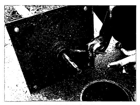
126. Again bituminous paint is added (to the thread on the underside of the pump stand and pump rod)
