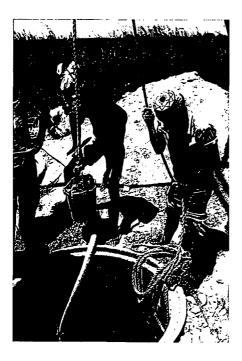
36. A bucket is filled with soil and pulled up
