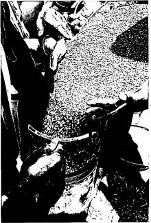
77. The filter material is poured between filter pipe and casing
