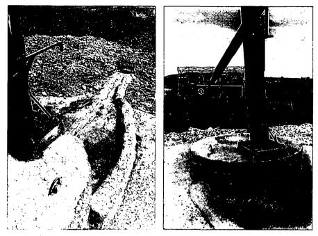
83. A gutter guides the spoil water to a drainage area
