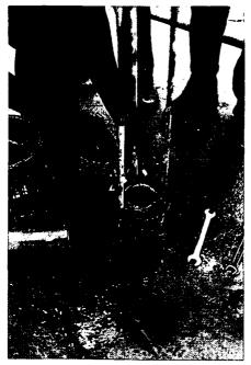
117. Bituminous paint is applied to the groove in the bottom flange
