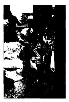
127. Pump rods are connected. (The lower one is fixed. The upper one is turned by turning the pump superstructure)
