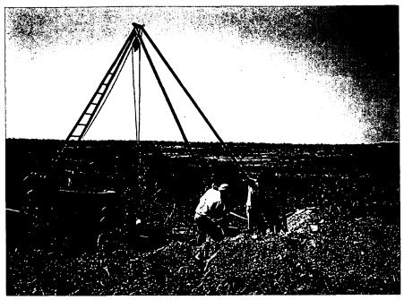
48. The tripod is repositioned so that the tackle is exactly over the centre of the well
