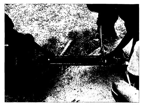
121. And the rising main and pump cylinder are connected
