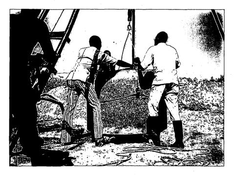
51. The guide-rope around the ring is repositioned to prevent askew lowering
