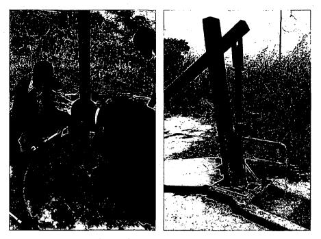
129. The footplate is bolted to the cover plate
