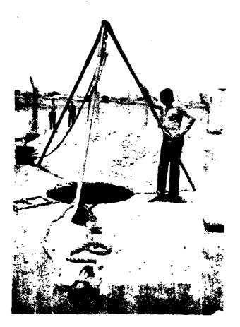
Figure 8-2. Bucket and rope.
