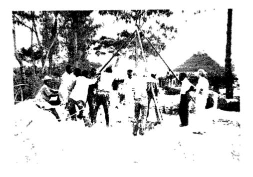
Figure 8-7. The well ring installation by using a tripod.
