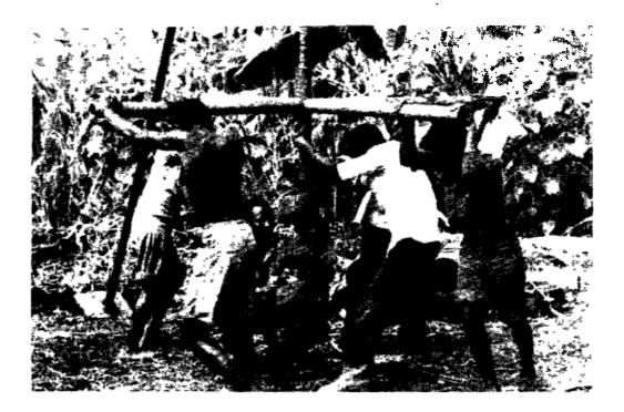
Figure 8-12. Hand drilling in operation in Morogoro.
