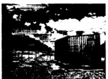
Fencing the pump house area helps protect the ground water from being polluted
