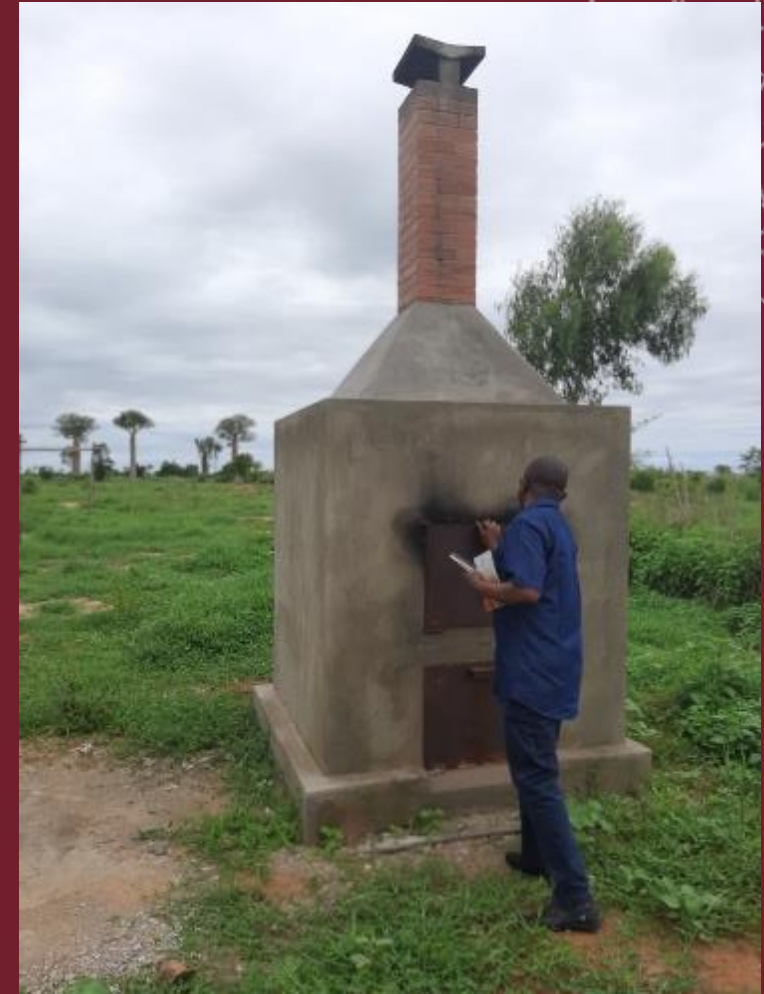
Single-chamber incinerator at Providence HC in Madagascar/Photo Francois, CRS
