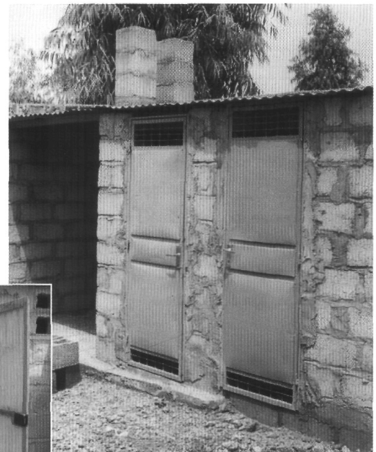
VIP latrines constructed in a planned peri-urban area.
