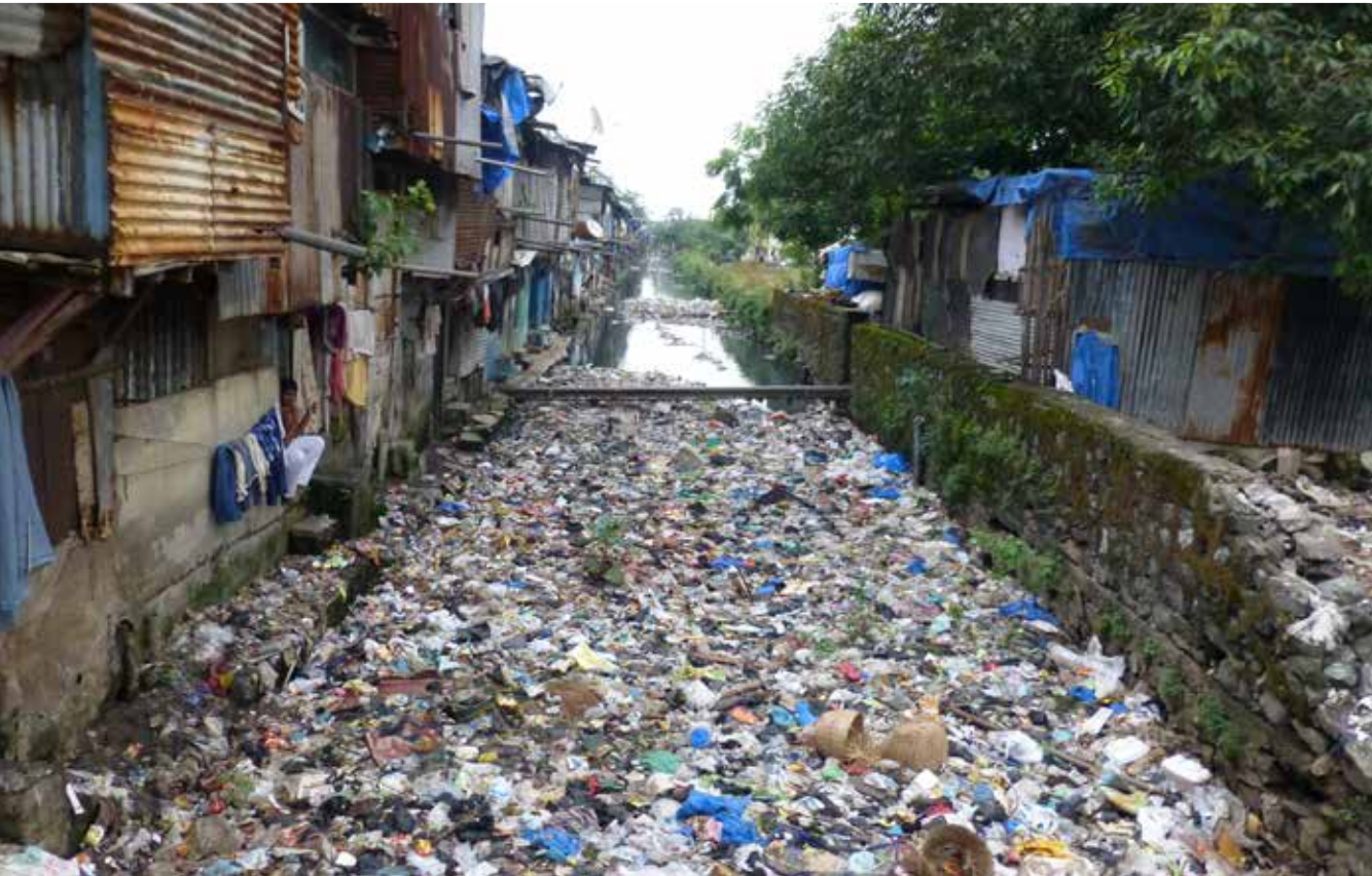
Convergence of human and solid waste in a stormwater drain in Mumbai, India (Photo by Giacomo Galli/ IRC).
