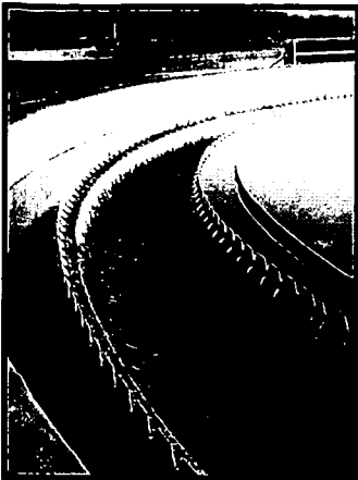
The existing sewage treatment plant for Hungary's second biggest city, Miskolc, which will be upgraded following the completion next year of a £10 million study and design project involving consultant Mott MacDonald.
