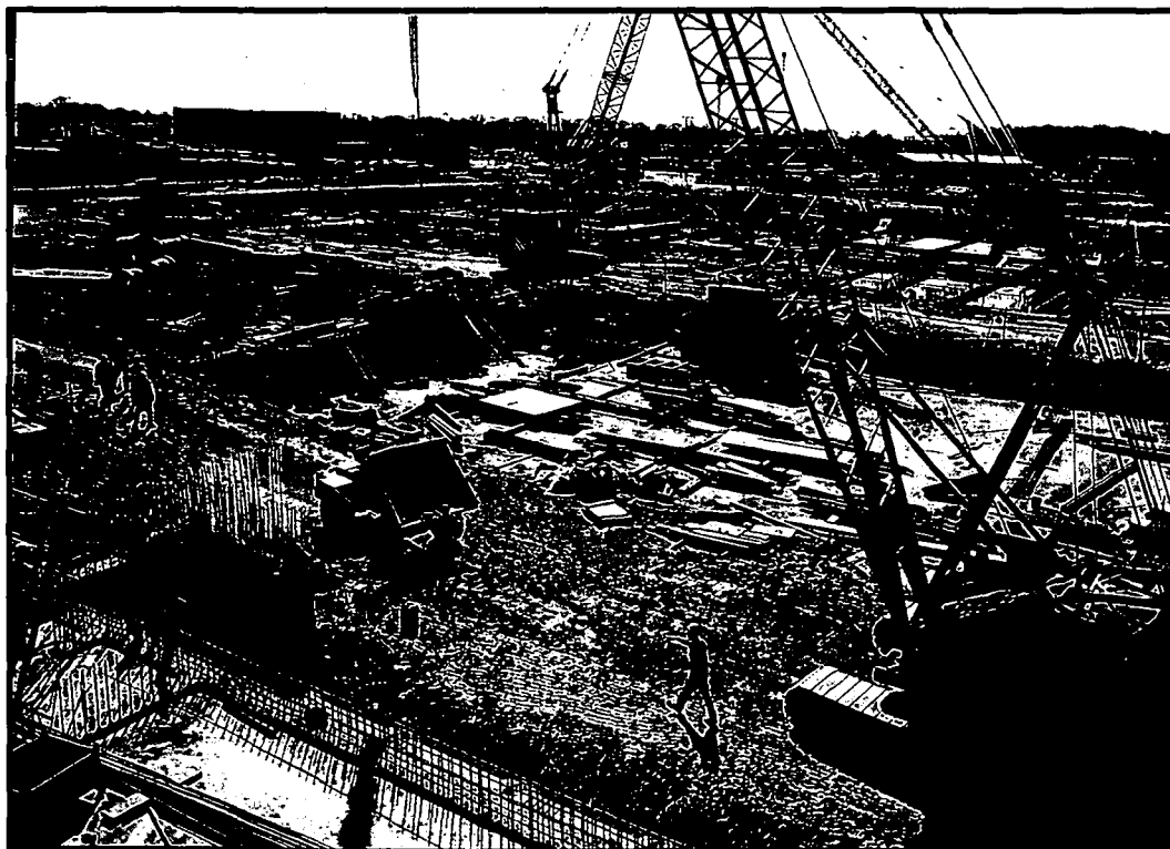
Construction of a £54 million project by Anglian Water claimed to be the most significant water-treatment plant in size and technology in Europe. Grafham will remove pesticides and herbicides from drinking water at 350,000 cubic metres a day
